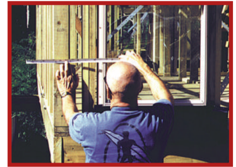
Setting windows and doors to suit brickwork
