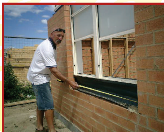
Determining Brick sill quantity
