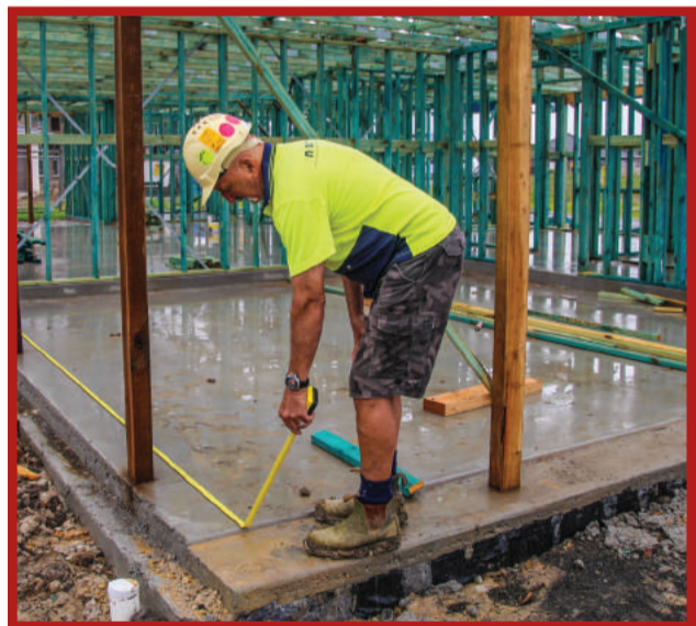
Establishing brick bond off a slab
