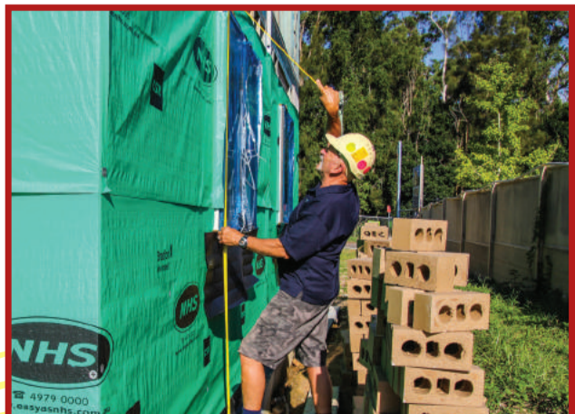
Set out window, door & arch bar heights from slab or footing for correct window and door position - no need to move them prior to the commencement of work!
