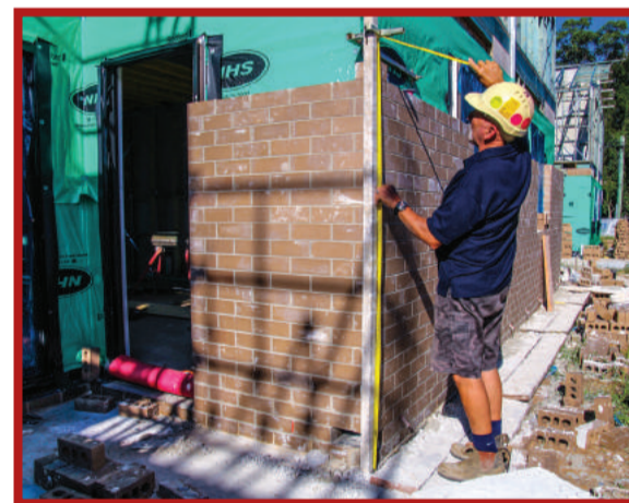
With numbered gauges 84, 85, 86 & 87 you can set out gauge from drop off point and eaves to footings and slab to check how many courses and whether you need to open or close the gauge - no more pigs!
